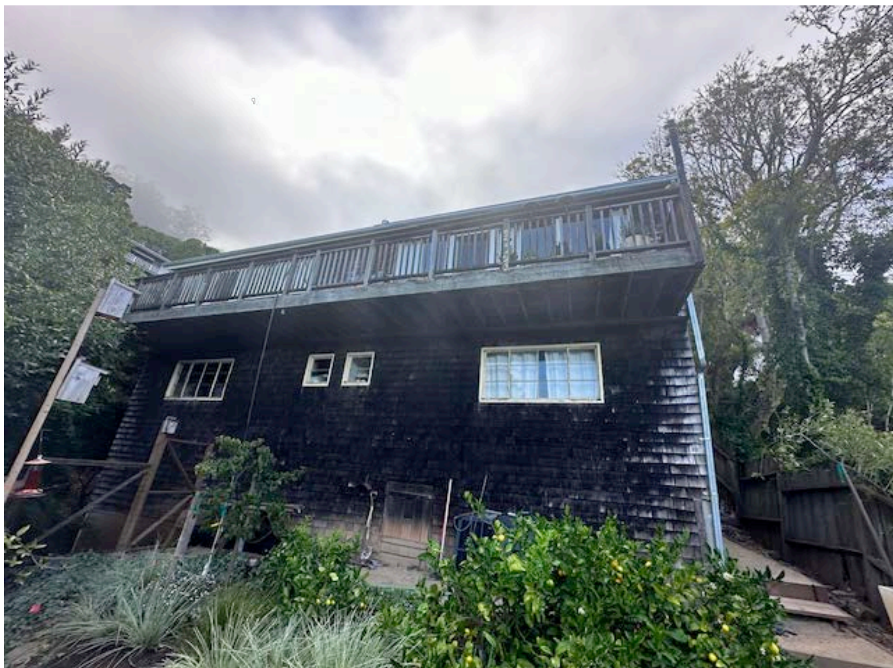
5 PHOTO EAST ELEV. (SIDE)
