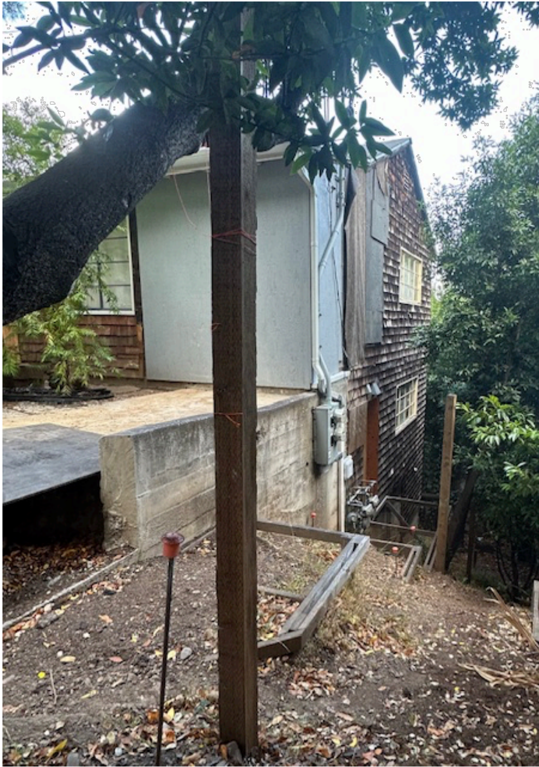
3 PHOTO - SOUTH ELEV. (SIDE)
