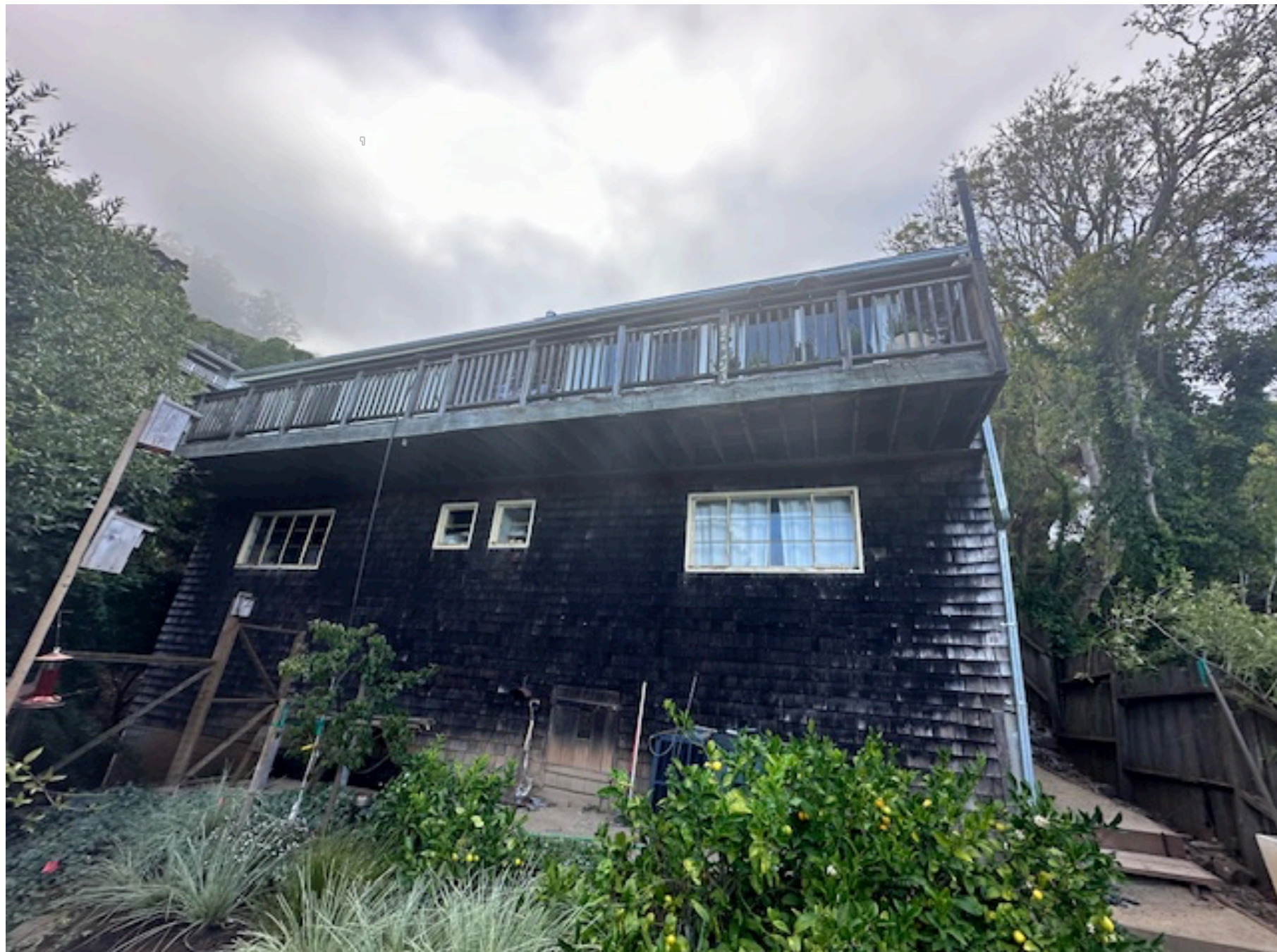
5 PHOTO EAST ELEV. (SIDE)
