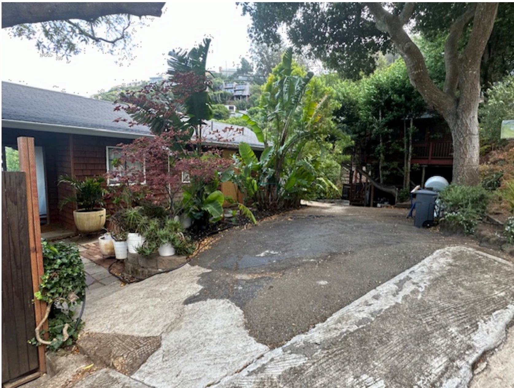
2 PHOTO - WEST ELEV. (FRONT) - LOOKING AT DRIVEWAY
