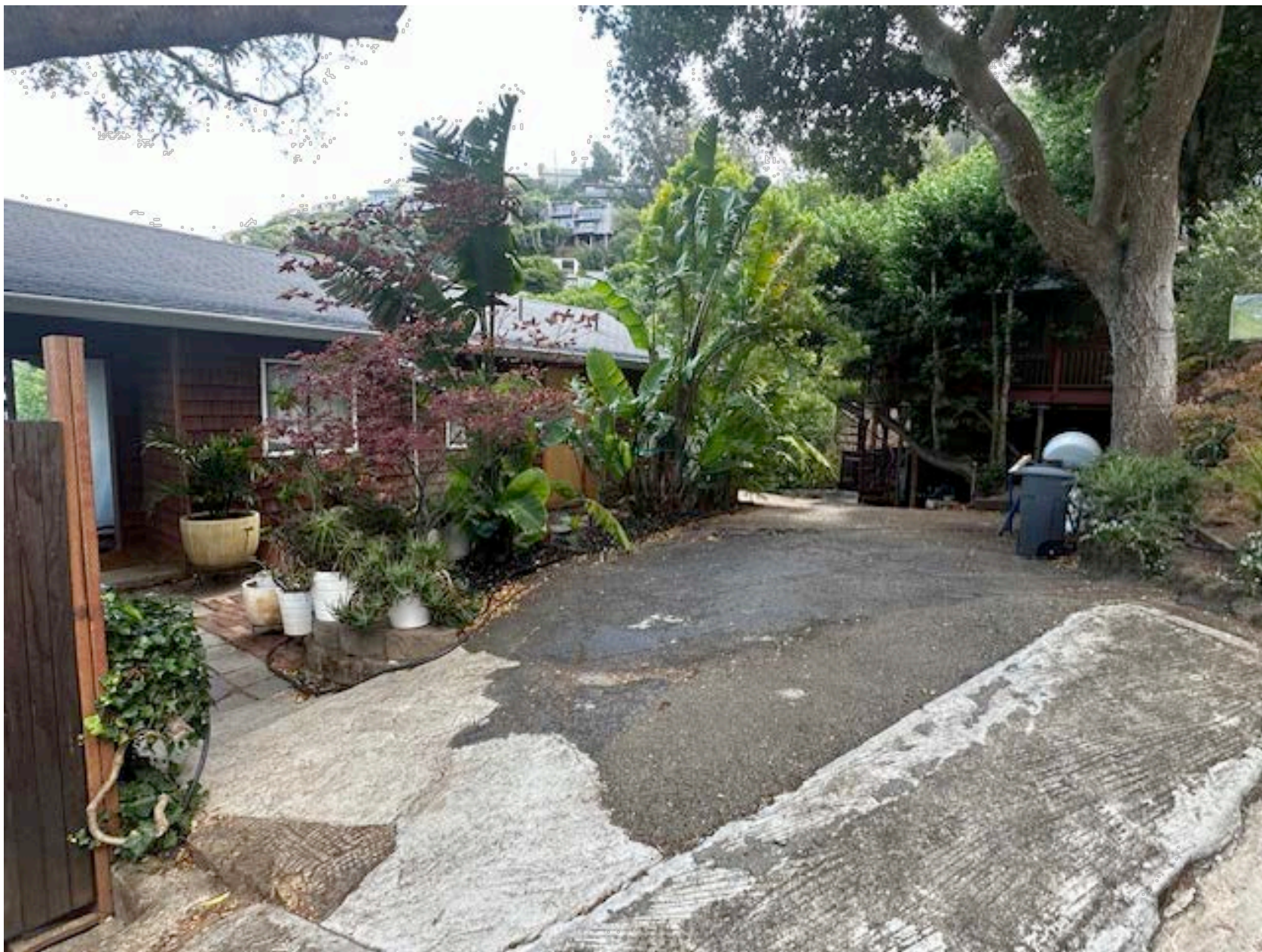
2 PHOTO - WEST ELEV. (FRONT) - LOOKING AT DRIVEWAY
