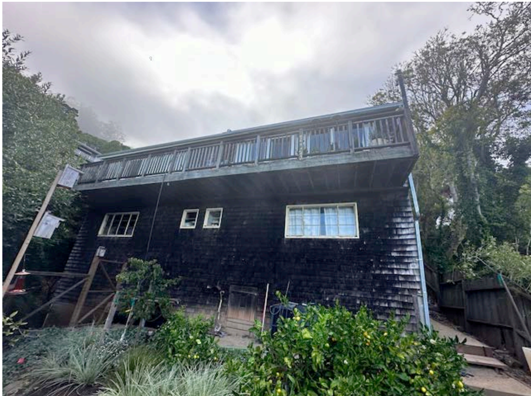
5 PHOTO EAST ELEV. (SIDE)
